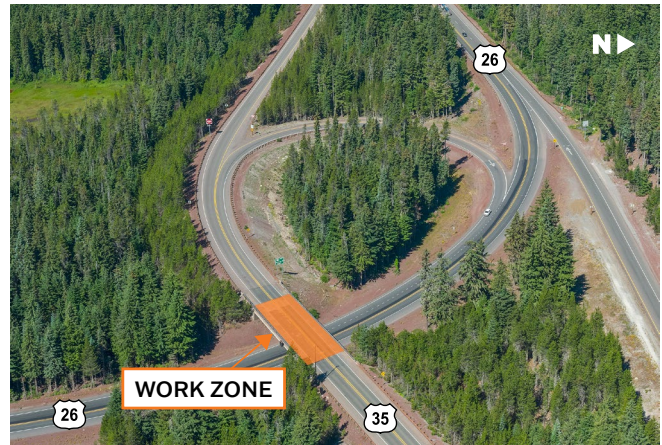
Aerial photo of project area, looking west.
